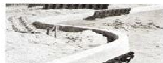
Full height segmented batter face plates are used.
