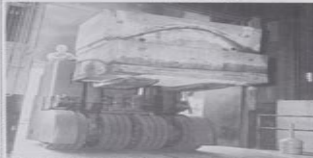
MONSTER—Newest addition to Convair Fort Worth's rolling stock is this 40,000-pound capacity lift truck. Here S. E. Allen of traffic men truck loaded with metal die as truck enters south end of plant. One of only three such in U. S., truck may be driven from either side with dual control. Largest lift truck at Convair SD has 20,000-pound capacity.
