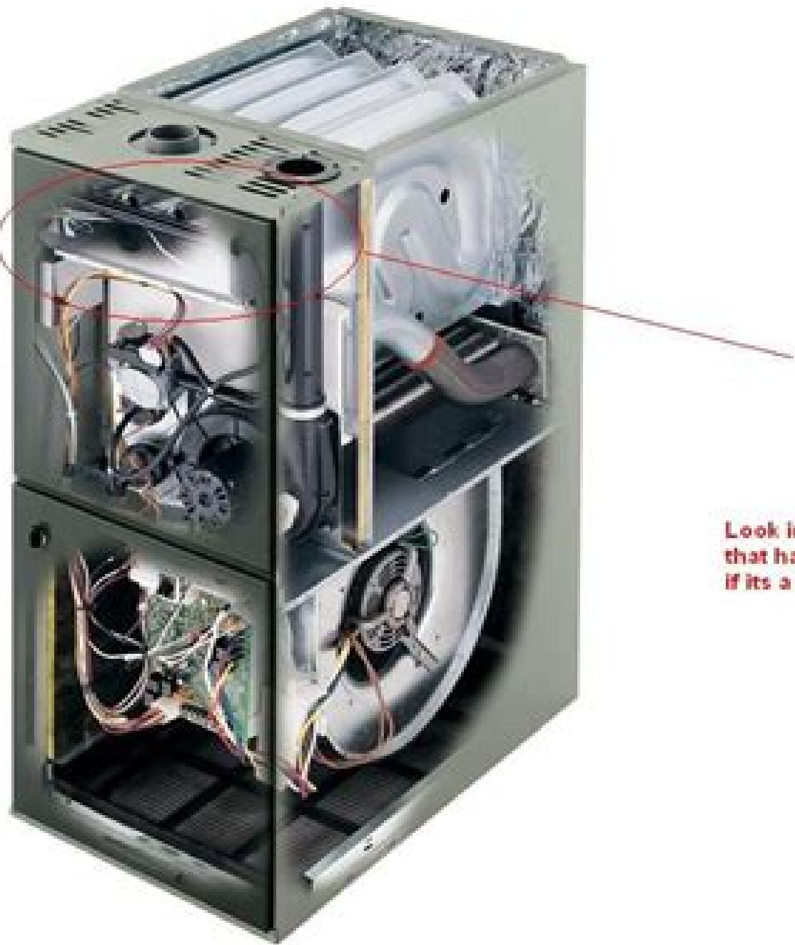
Look in this area for a rollout switch that has a button on it, reset it there if its a limit rollout problem.
