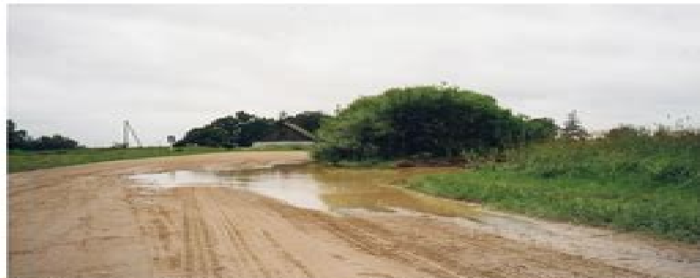
Lack of a roadside ditch has caused major drainage problems on this road. (Courtesy of Road Research Ministry of Roads/Transportation, Sweden)
