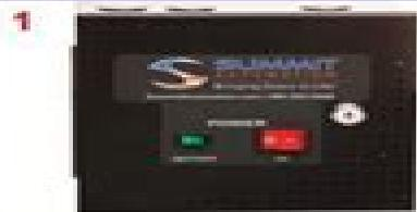
1. Turn the red AC power switch off and the green battery switch off, located on the exterior of the control box. Move the door into the fully closed position.
