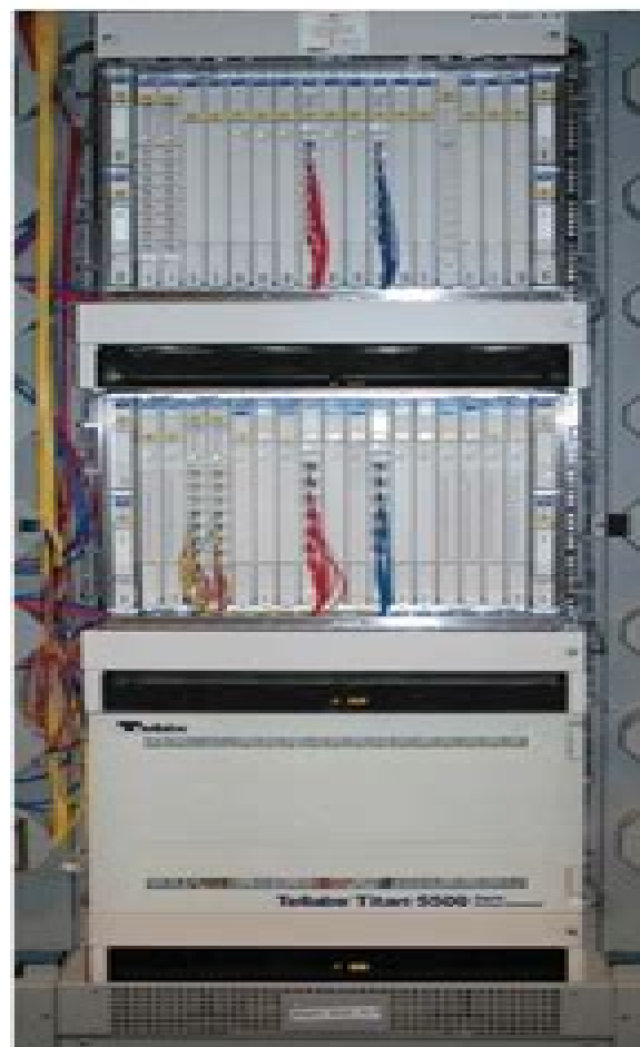
Tellabs® Titan® 5500 Digital Cross-Connect shelf
