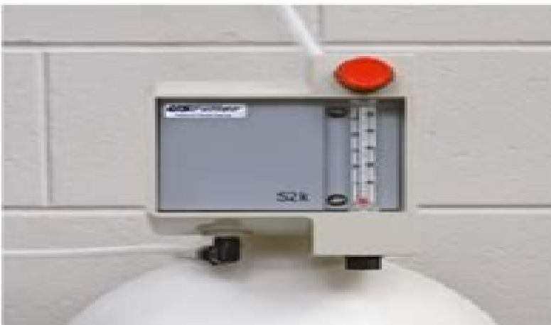
water supply and running plastic tubing to a main or open channel. A knob adjustment changes gas feedrate, which is indicated on a 3-inch-scale rotameter. The insertion need not be shut off when changing cylinders. Maintenance requires only a wrench and a screwdriver.
